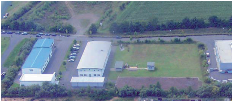
EBINGER Technology centre Wiesbaum
